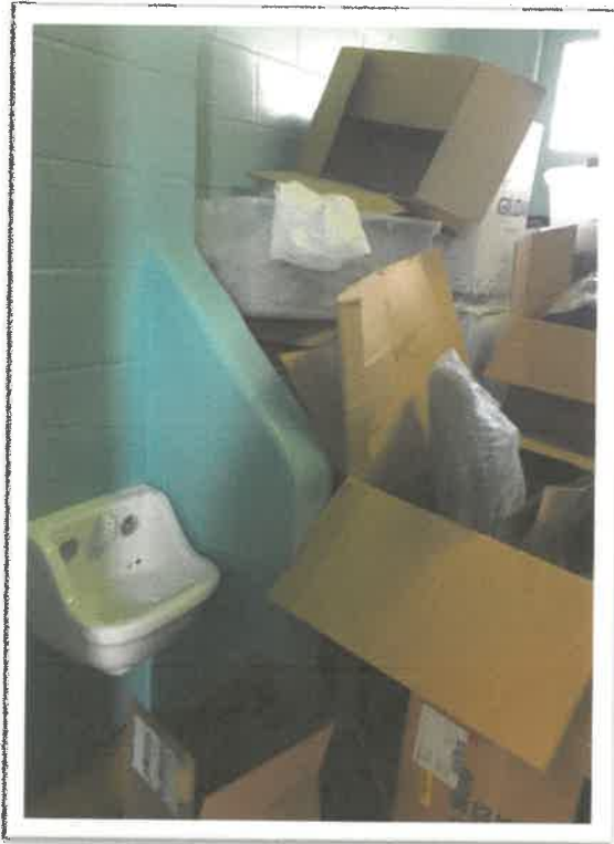
Photo F- Mod 1 Room used for Storage
